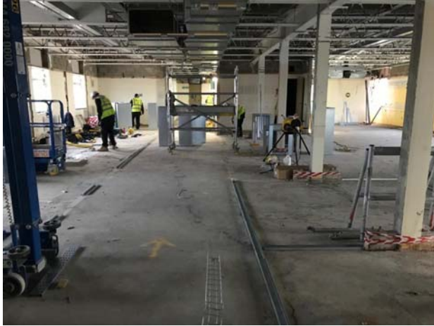
Fig 2: Internal view of the ward refurbishment work
